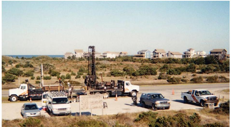
*Roto sonic-drilling rig set up adjacent to dunes south of Avon, NC.*
