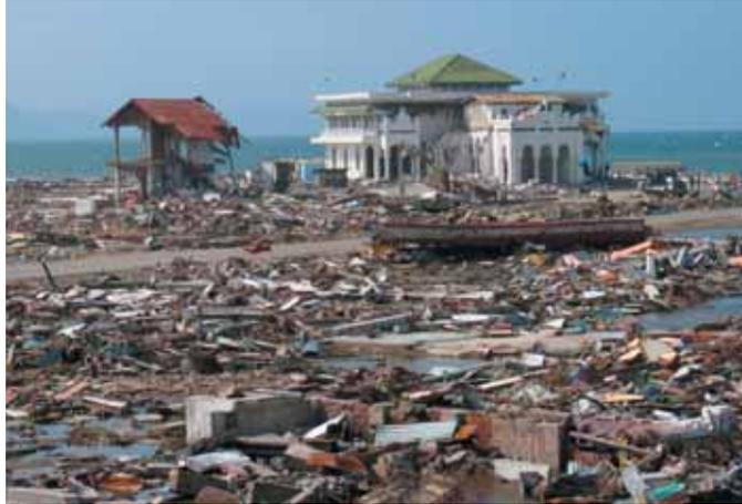
*A mosque is left standing amid the rubble in Banda Aceh. Several mosques survived and may have been saved by the open ground floor that is part of their design. The tsunami waves reached the middle of the second floor. Photograph by **Guy Gelfenbaum**, USGS.*
