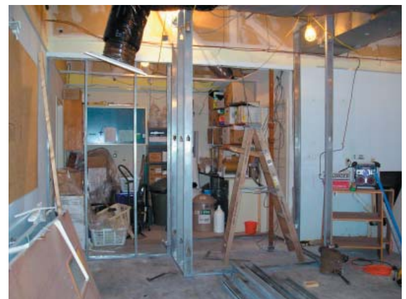
A view of the larger clean room undergoing renovation. The facility will have two rooms, the larger at Class 100,000 and the smaller at Class 10,000. The total area of the facility will be 500 ft 2 . Photograph by Sarah Kelsey .
