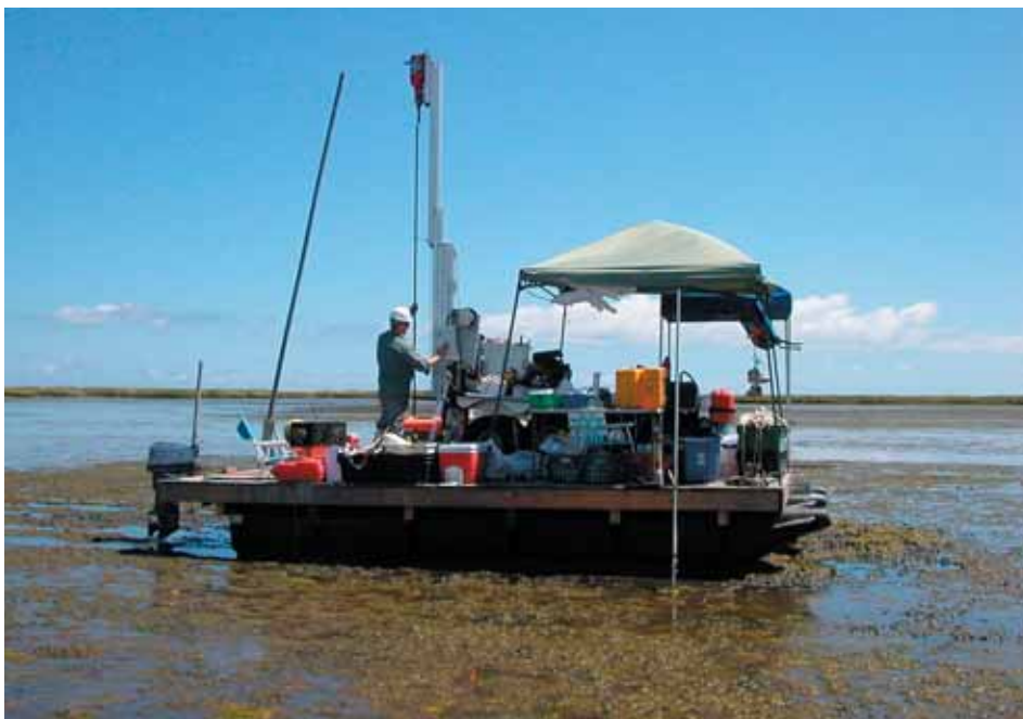
Andy Massey (USGS) operates a drilling barge that is temporarily stranded during low tide on a mudflat at Cape Cod National Seashore.
