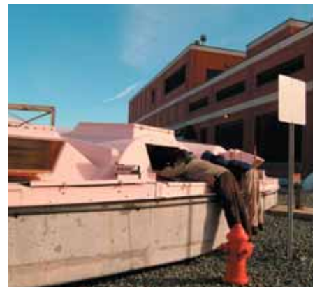
This diffuser on display at the Deer Island Sewage Treatment Plant is like the 55 diffusers that are underwater along the last 1.5 miles of the sewage outfall tunnel, which extends 9.5 miles eastward from the treatment plant and Boston Harbor into Massachusetts Bay. Photograph by Dann Blackwood .
