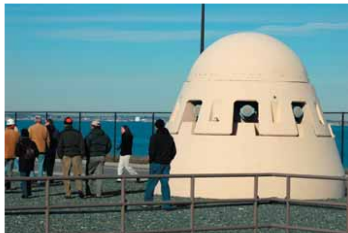
► Dann Blackwood and Tim Milbert peering into a gravity thickener used to consolidate the sludge from primary treatment for later digestion in the egg-shaped digester tanks. Photograph by Sandy Baldwin .
