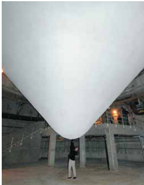
Sandy Baldwin standing underneath one of the digesters, or "eggs," holding 3 million gallons of sludge. Photograph by Dann Blackwood .
