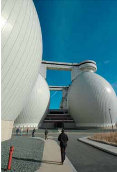
A few of the 12 egg-shaped digesters using heat and microorganisms to break down solids and toxins from the effluent at the Deer Island Sewage Treatment Plant. Photograph by Dann Blackwood .
