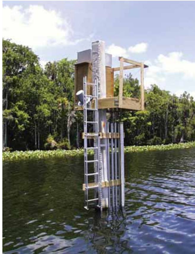
Stream gage at the Suwannee River above the Gopher River near Suwannee, Florida (7.6 mi upstream from the mouth of the Suwannee; see map, p. 3). The metal box on top of the wooden platform houses the DCP and battery. Water level is measured by a pressure transducer in a polyvinyl chloride (PVC) pipe—a “stilling well” that isolates the measured water surface from waves and ripples (pipe is hidden by concrete pillar in this view). Data are transmitted to the satellite through a GOES antenna attached to the wooden platform (behind left side of ladder, shaped like a top hat). Photograph by John Pittman, November 3, 1999.
