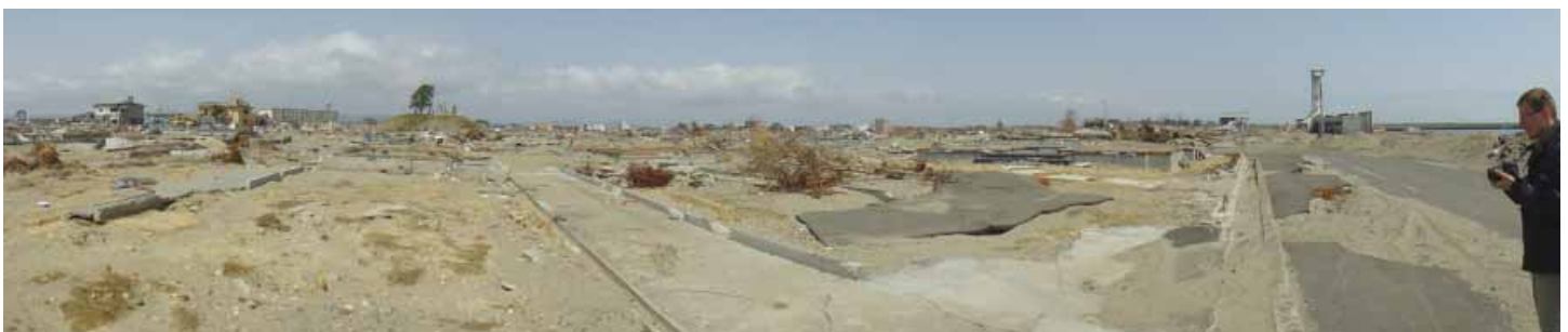
The March 11, 2011, tsunami destroyed most buildings in Yuriage, leaving exposed foundations and scattered debris. The tsunami flow was about 8 m (26 ft) deep here and moved a stone monument off the top of the artificial hill in the background on the left side of the photograph. The stone had been placed as a reminder of the 1933 Showa tsunami that killed many in Yuriage.
