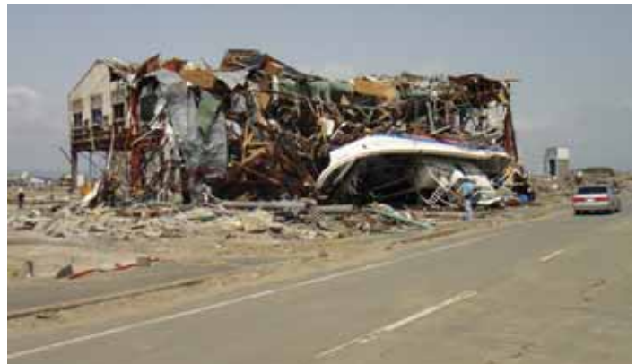
Building damaged by the tsunami in Yuriage. The tsunami flow depth here was approximately 8 m (26 ft).
