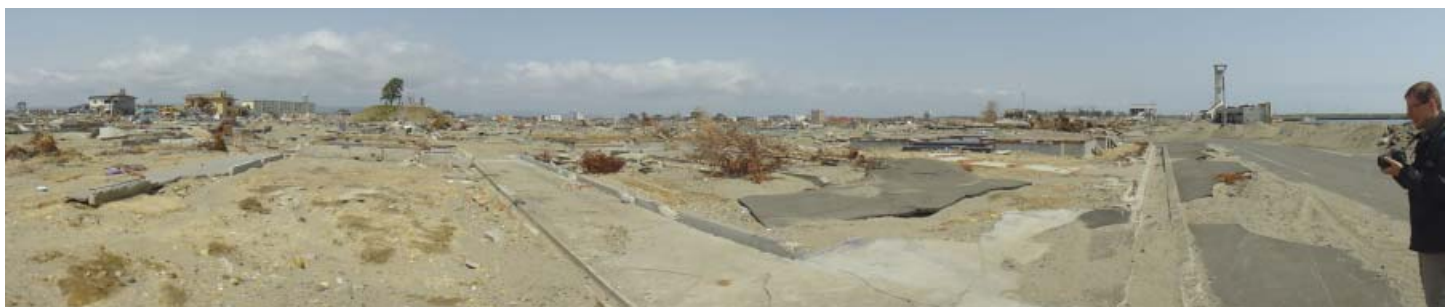
The March 11, 2011, tsunami destroyed most buildings in Yuriage, leaving exposed foundations and scattered debris. The tsunami flow was about 8 m (26 ft) deep here and moved a stone monument off the top of the artificial hill in the background on the left side of the photograph. The stone had been placed as a reminder of the 1933 Showa tsunami that killed many in Yuriage.
